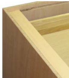
Particleboard construction (side detail)
