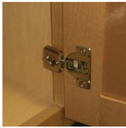
6-way Adjustable hinges (standard overlay detail)
