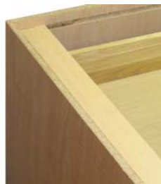
Particleboard construction (side detail)
